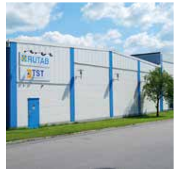
Warehouse - and production facility in Nässjö, Sweden
