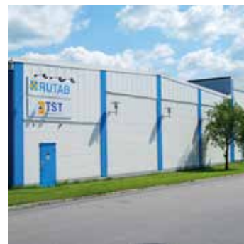
Warehouse - and production facility in Nässjö, Sweden
